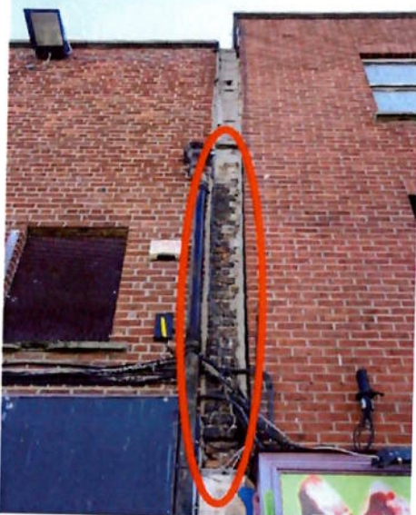
Fig. 5: Retained two-storey section of historic party wall (encircled red) between the modern new-builds at 12 (RHS) and 13 (LHS)
